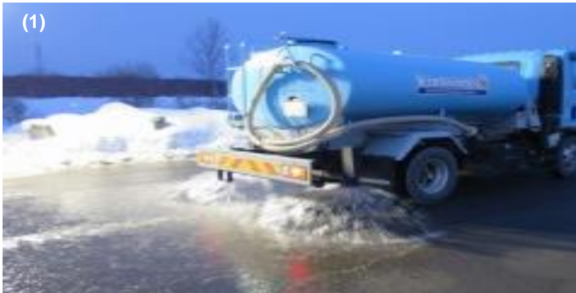
Sprinkling water for making ice film on the surface
